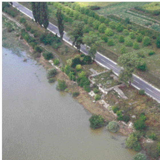
70. The massive stone blocks of a smaller bridgehead of the late Roman period are situated on the left riverbank close to Nógrádveroce (Hungary)
