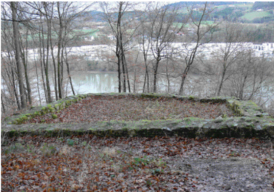
64. Excavations in the woodland above the Danube at the watch-tower of Hirschleitengraben in Upper Austria have brought to light an older structure dating back to the 2nd century AD
