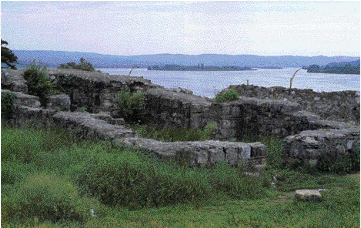
128. The Roman fort at Drobeta close to the modern town of Turnu Severin in Romania was built on the left bank of the river Danube as a bridgehead into Dacia
