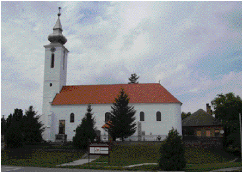
116. Roman masonry and stone monuments are visible at the outside of the church at Lug (Croatia)
