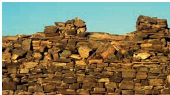
104. Crenellations at the fort of al-Zarka Créneaux du fortin d'al-Zarqa
