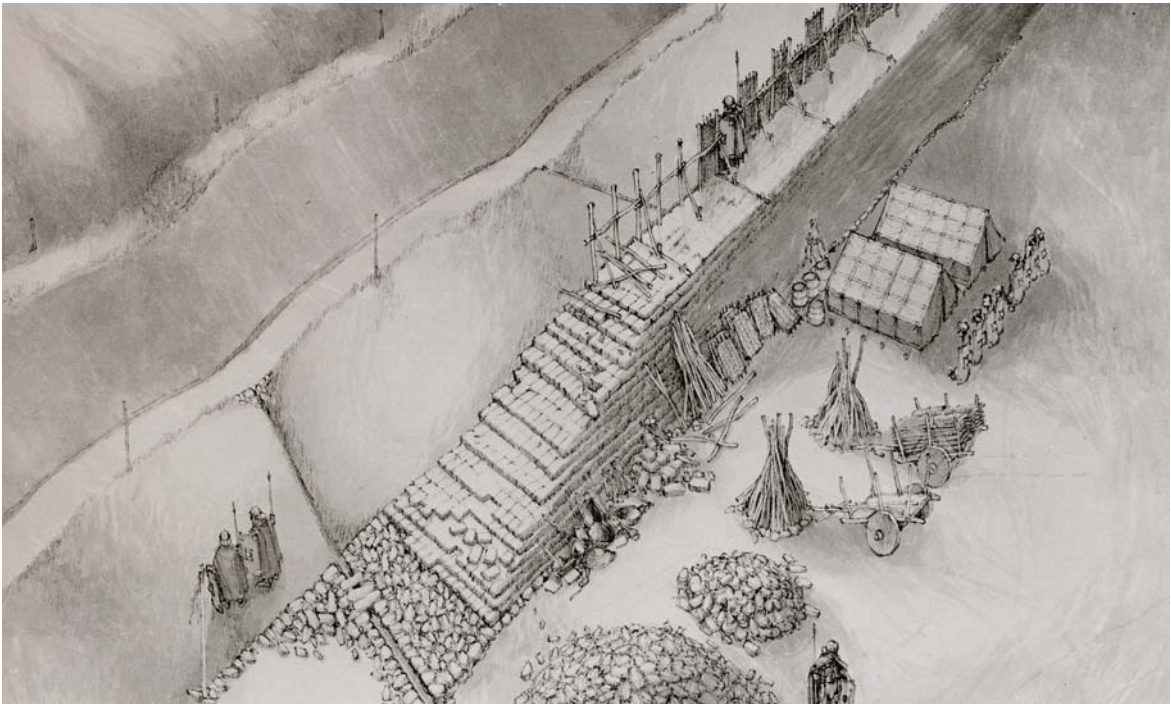
79. An artist's impression of the building of the Antonine Wall. This illustrates several activities which would not have taken place at the same time: the laying of the stone base, the placing of the turf blocks, cut to regulation size 18 by 12 by 6 in, and the construction of the breastwork, assuming one existed (drawn by M.J. Moore)
