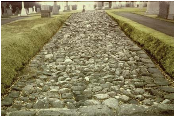
66. The stone base of the Antonine Wall in New Kilpatrick Cemetery, Bearsden. The base, 15 Roman feet (4.3 m) wide, is crossed by a drain
