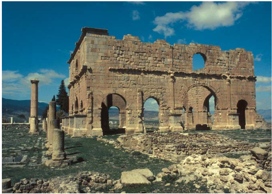
35. The remains of the headquarters building of the legionary fortress at Lambaesis (Algeria) Die Überreste des Hauptquartiers des Legionslagers in Lambaesis (Algerien)
