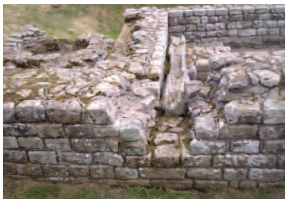
104. A channel brings water to the soldiers at Chesters. An oven lies beside the tower
