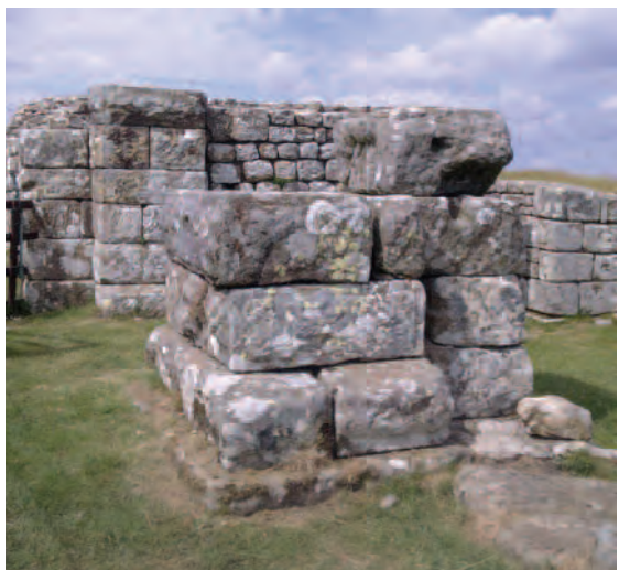
90. The west gate at Housesteads with the upper stones less well dressed than those below
