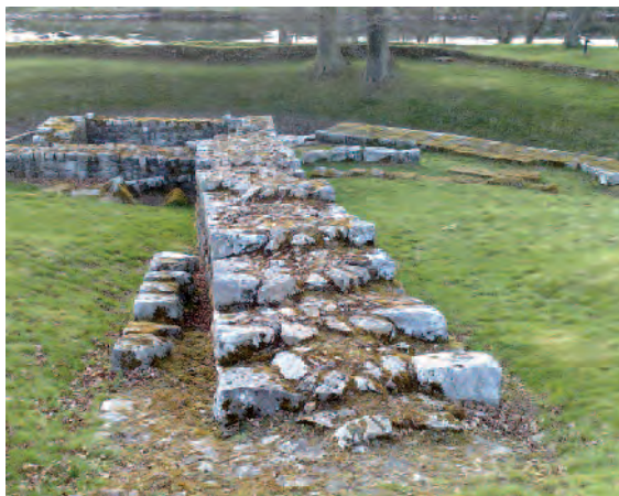
88. The Wall at Chesters bridge abutment showing the earlier foundation to the south
