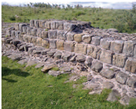
89. Different stages in building of the Wall: broad foundation, narrow foundation and narrow wall
