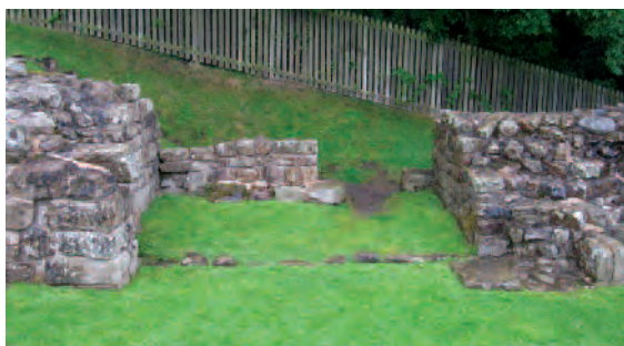
103. The north gate at milecastle 48 (Poltross Burn) was narrowed, like many such gates
