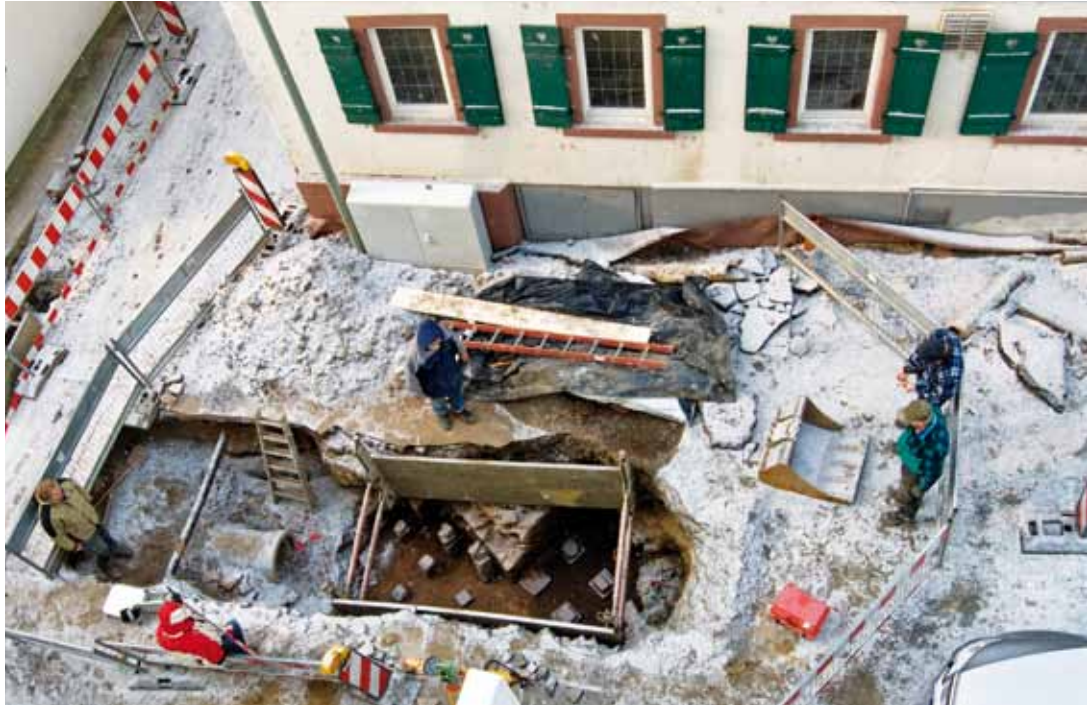
Bad Ems. Rescue excavation of the bath buildings in front of the fort.
